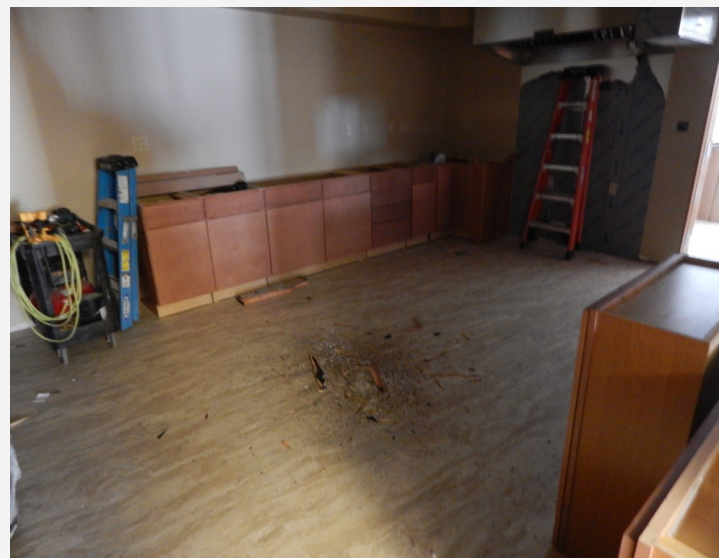
Kitchen with new flooring and cabinets going in
