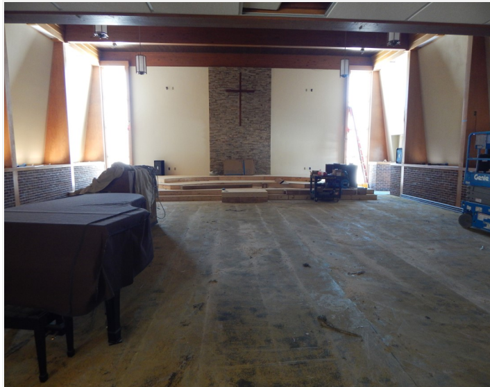
Sanctuary with new front windows and ready for new carpet
